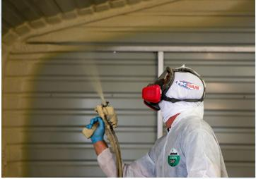
Profoam offers a wide range of SPF products which are available in various densities, each exhibiting different performance characteristics such as moisture resistance, R-value, and structural properties. In the case of metal buildings, closed-cell foam is typically used due to its moisture control and structural characteristics.
